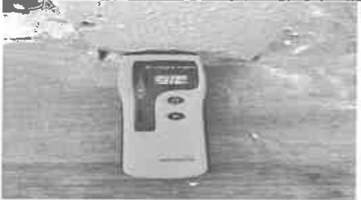
Laundry/ utility room- WME 20.9% at closet wall where hot water tank is located
