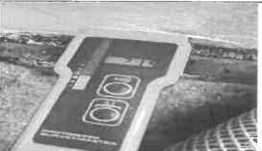
Living room- WME 21.9% at 1.5 ft mark at wall base
