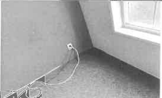
Living room wall where the laundry/utility room share a wall
