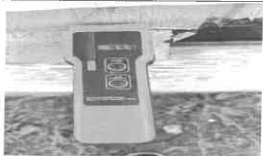
Exterior wall at laundry/utility room-WME 100%
