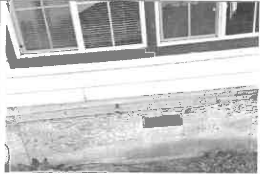
Exterior wall at living room
