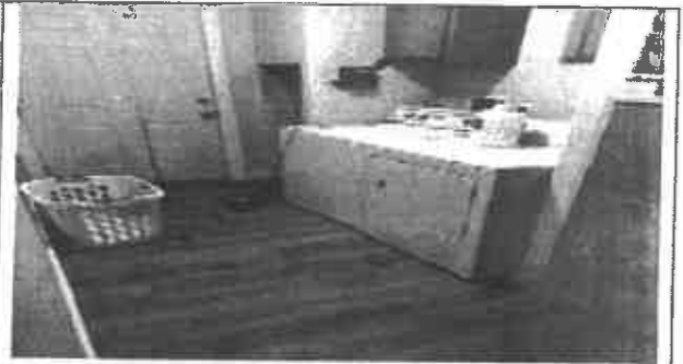
Sample # PCFD -PRV - 2 Laundry/Utility Room
