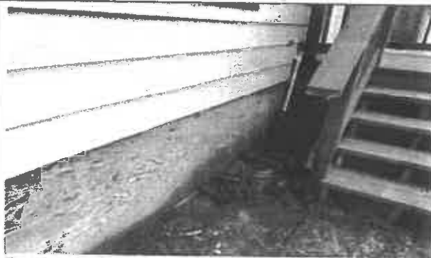
Compromised skirting and siding replaced: good now
